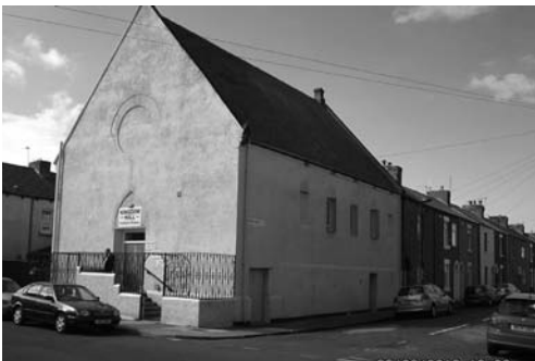
Wallsend Co-op School now Kingdom Hall Blenkinsop Street Wallsend
